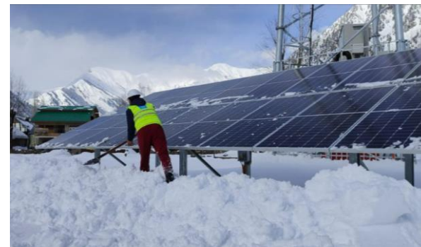
Site operations during heavy snowfall
